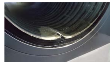
Fig. 3. Fracture of the end
